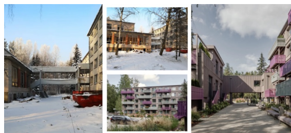
Figure 8: Edinburgh Apartments & Lofts project, designed by OAD. Source: https://oad.archi/work/edinburgh
